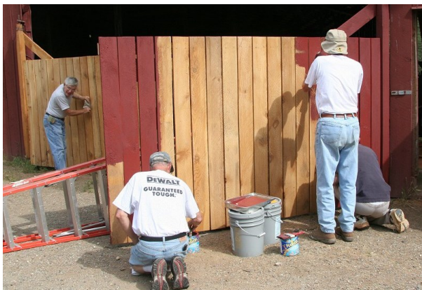
Volunteers putting fresh paint on the historic barn.
